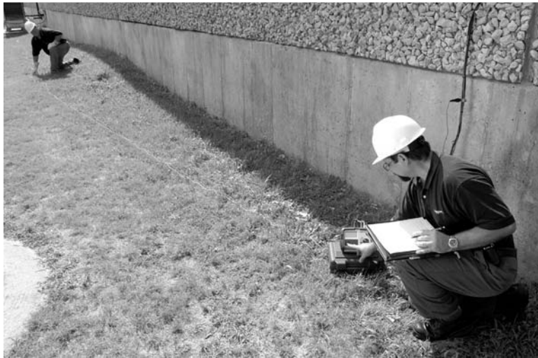
Ground test being performed on building ground using a DET3TC
